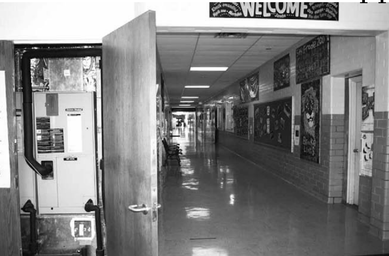
Heating, Ventilation and Air Conditioning Renovations at Brooke Elementary School
